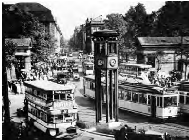
Figure 1: One of the first electric traffic lights in Germany: Installed in 1924, the five-edge semaphore tower in Berlin was equipped with lamps from Siemens operated by hand by policeman in the tower
