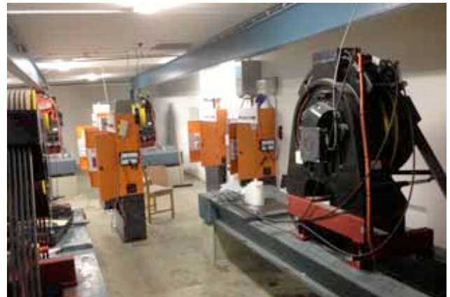
Figure 1: View of engine room during modernization
