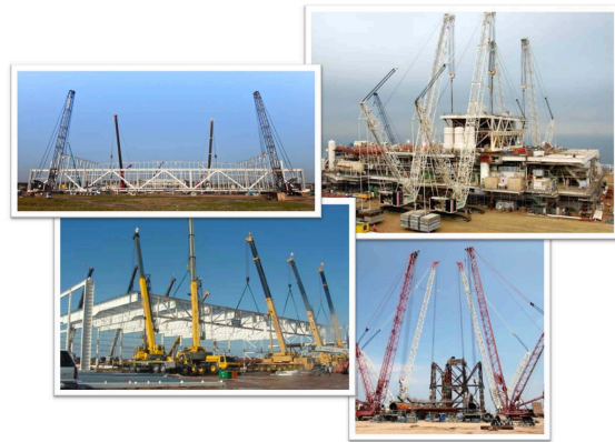
Figure 12: Wireless communication supporting multi crane lift jobs
